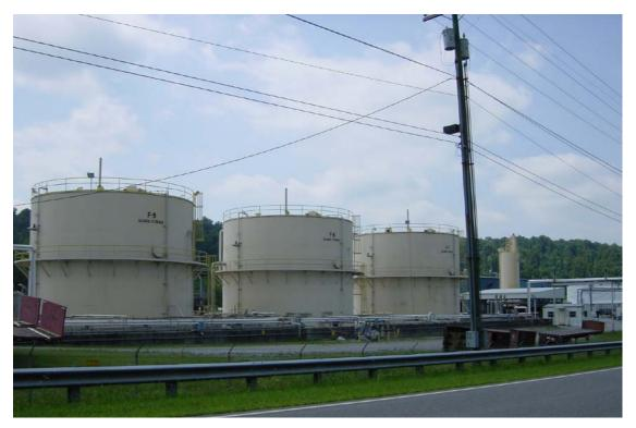
A US Department of Energy used four 500,000-gallon AWW Water tanks to store sludge through the 1940's and 1950's. The tanks were not originally designed to store sludge since they had a flat, rather than a conical, bottom.
