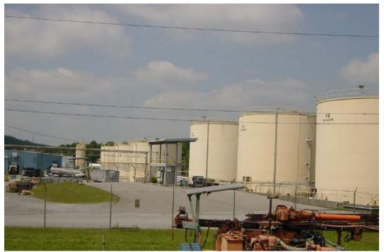
The tanks had 8" flanges with blanks located around the bottom circumference of the tank about 12" from the bottom. Taps of 4" diameter were run into the tank at multiple locations and liquid was removed. Positive displacement diaphragm pumps (air pressure) were used to pump the sludge.
