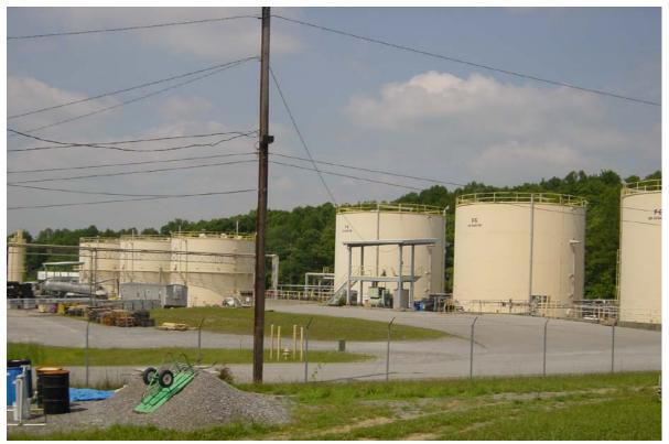
Three of the tanks had aqueous sludge waste with roughly 40-50% solids with radiation levels of 3000-4000 picocuries/gram. There was no external dose hazard from the tank.
