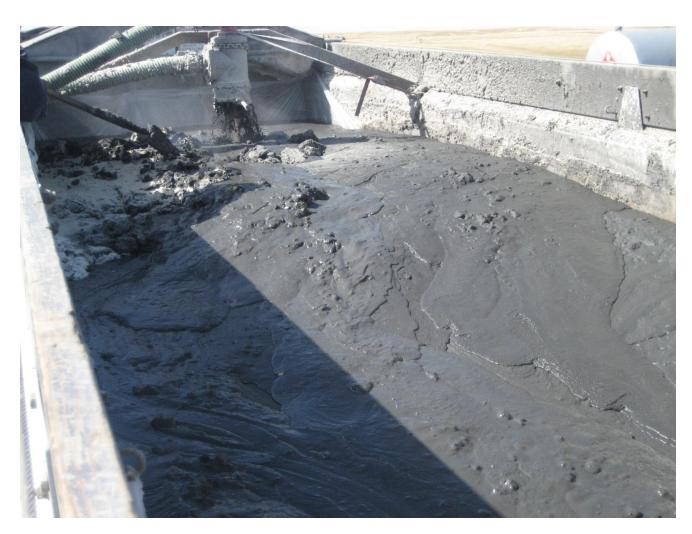
The truck rapidly fills up with stabilized sludge combined with sorbents.
