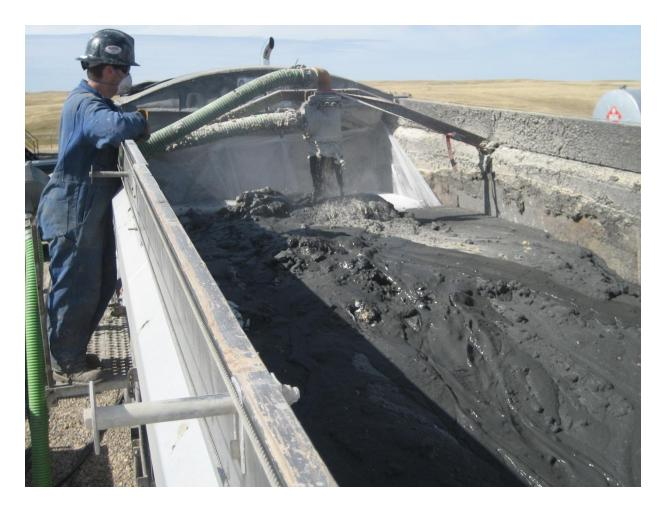
The water in the sludge is rapidly absorbed and the waste quickly loses flow ability of a liquid.
