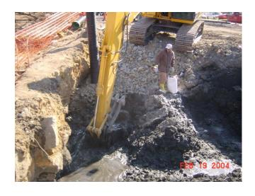
More sludge is added to top of polymer/sludge mixture.
